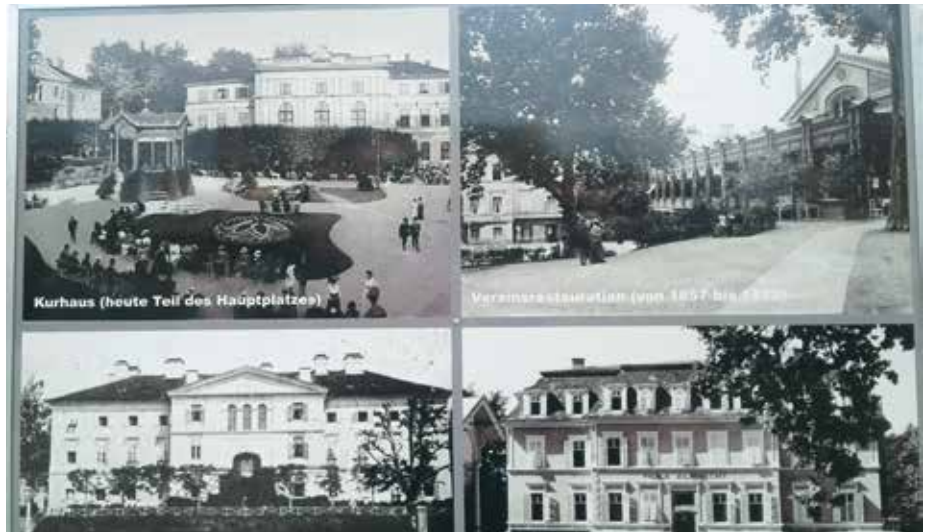
Bad Gleichenberg, historical photos (c) Ria Mang
